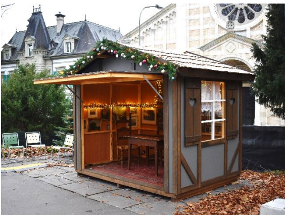
Framework style with shutters, glazing bars and shingle roof
